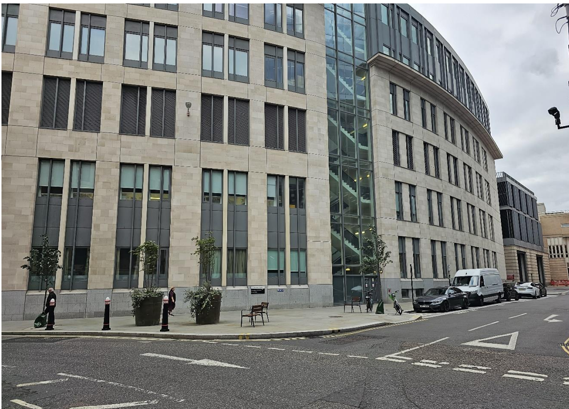
Phase 1 Area: Completed | Little Britain looking north from Montague Street
