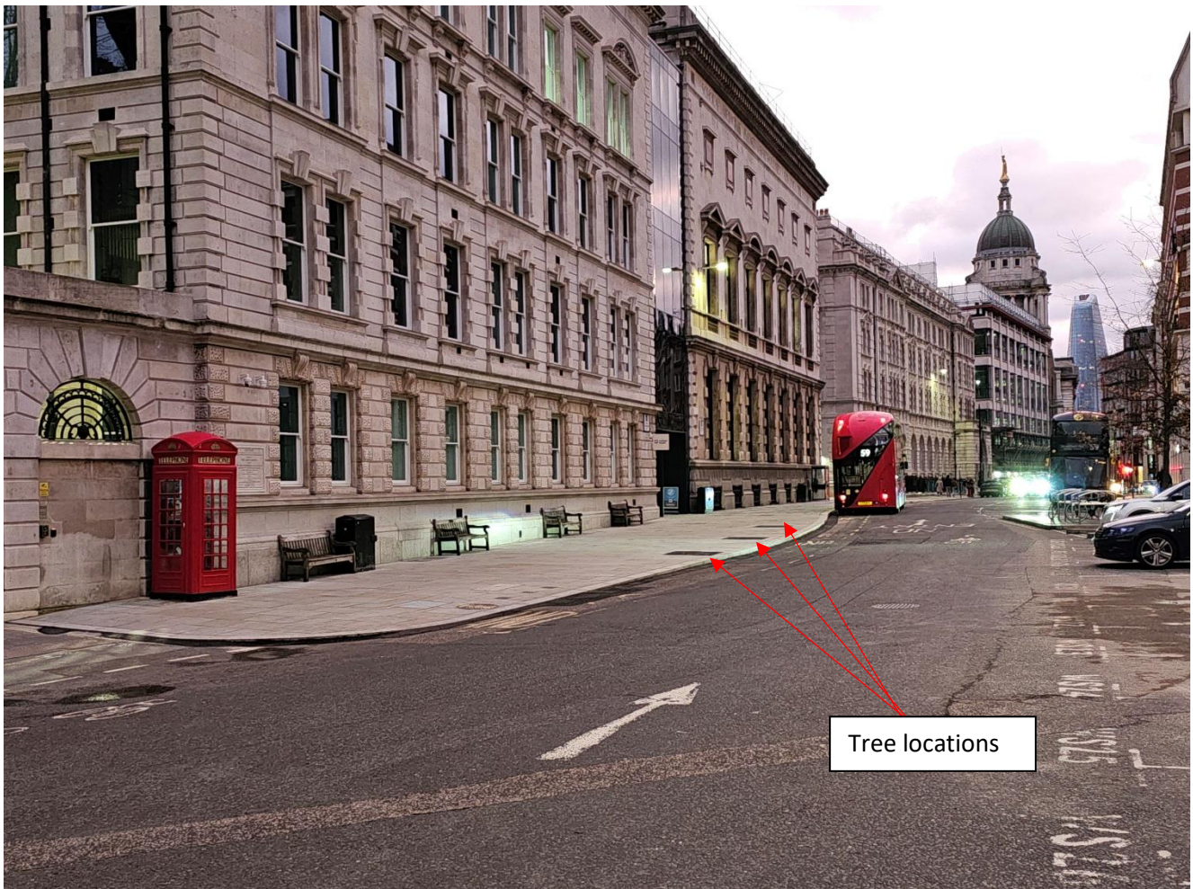
Phase 2 Area: Footway works largely complete, 3 Trees to be planted January 2024
